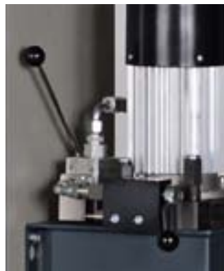
Detail of the two way valve selector (left) and loading/unloading valve (right).
