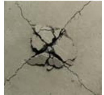
Typical failure under concentrated load
