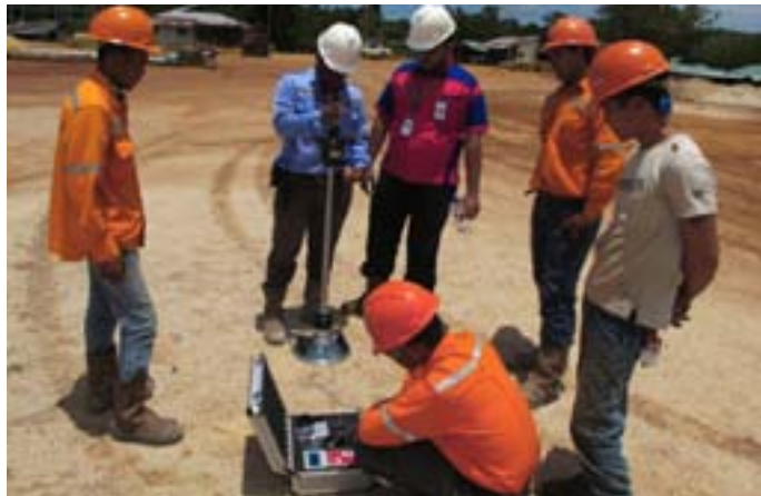
35-T0120 during operation
