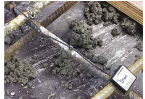
Installation Example of HG-4040
